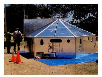
The Hexayurt is a simple, free, generic open source appropriate technology shelter which is designed to replace tents in many applications. Its unique feature is that it can be mass produced from a wide range of materials in simple or even improvised factories, or field-fabricated in about an hour with semi-skilled labor.
