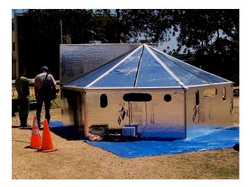
The Hexayurt is an extremely simple disaster relief shelter which is designed to replace tents in many applications. Its unique feature is that it can be mass produced from a wide range of materials in simple or even improvised factories, or field-fabricated in about an hour with semi-skilled labor.
